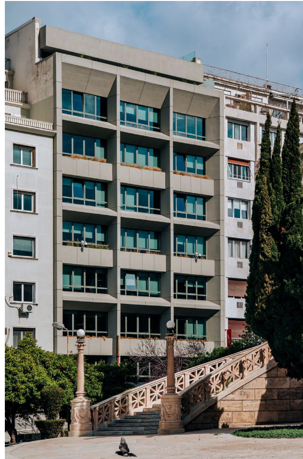
Remodeling of a multi-storey office building in the center of Athens
